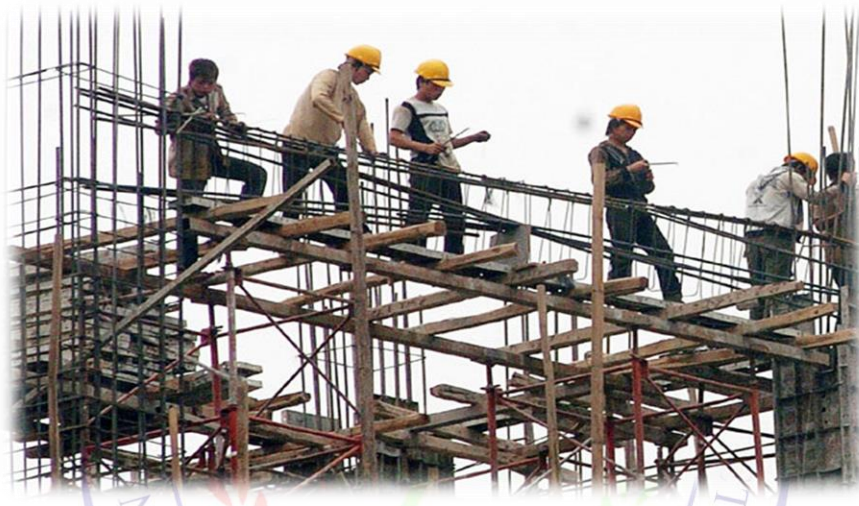
Fig. 2, Workmen working at height without ensuring fall protection safety measure, Sources Cons.
