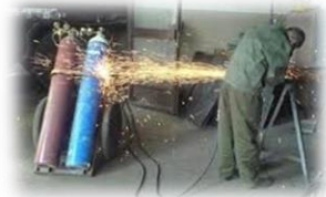
Hot Job near Combustible materials/ Fuel (C 2 H 2 /LPG) cylinder
