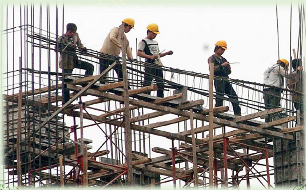
Fig. 2, Workmen working at height without ensuring fall protection safety measure, Sources Cons.
