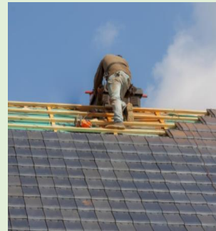
Potential of Fall from roof
